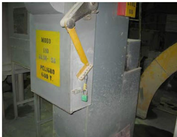
Fig 3 Lock out applied but no tag
