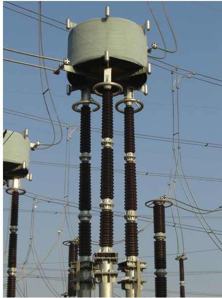
Figure 8: Wave Trap
