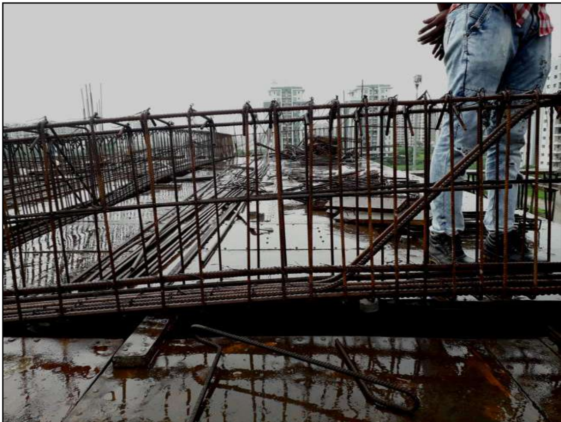
(Reinforcement Details of Beam)
