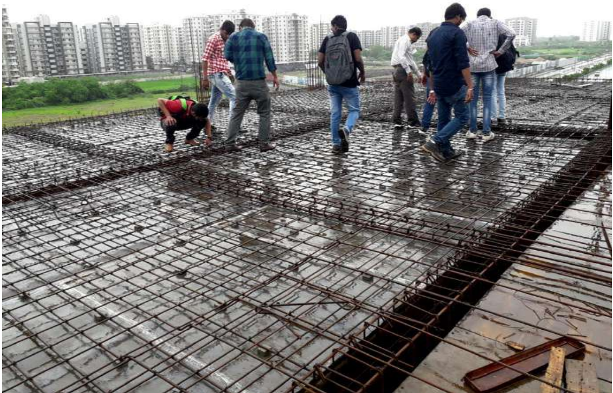
(Reinforcement Details of Slab)
