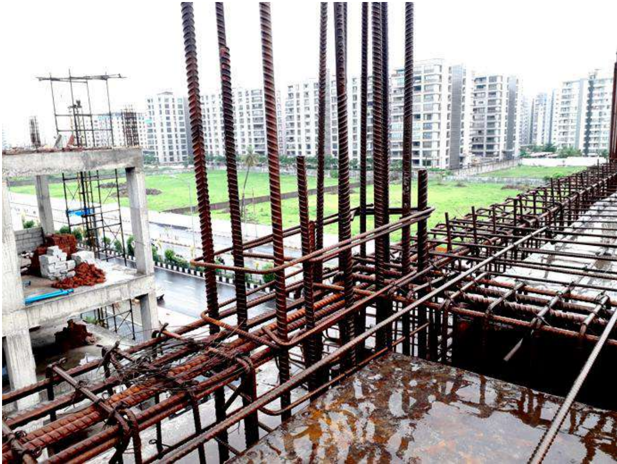
(Reinforcement Details of Beams and Columns)
